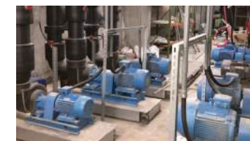
Air-conditioning chilled water pipeline replacement
