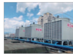
▲ Update the cooling tower in office buildings
