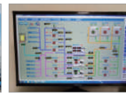
▲ Install air-conditioning environment control system
